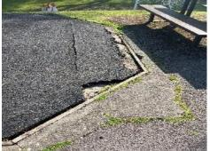
The cone is where the damage is. You can see the separation gap all around the area and where it has been patched before. The photo on the right-hand side shows the recent damage and bits missing.
